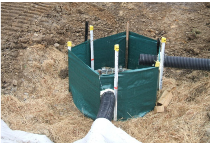
Good use of a silt fence installed to protect a new stormwater catchpit where impounded water will not create a flooding hazard
