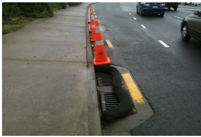
Installation of a silt sock to provide some protection to the catchpit
